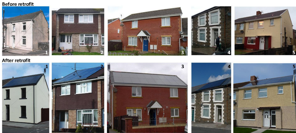
Demonstration LCRI Housing Retrofits (ERDF funded)
